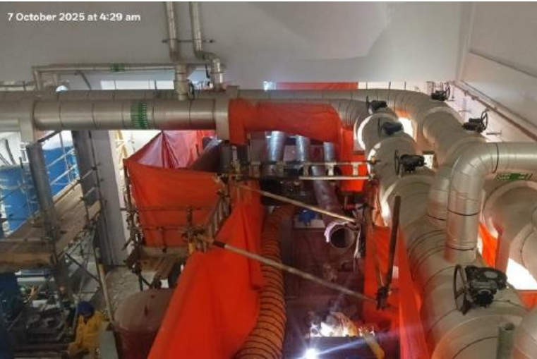
Chilled water pipe installation
