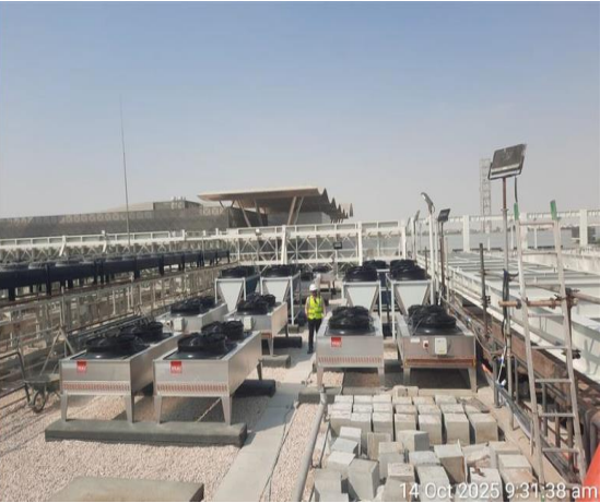
Condenser installation
